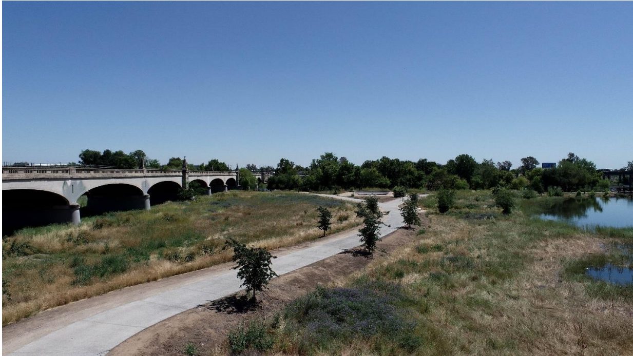
Figure 1. Existing Recreational Amenities – Trail View
