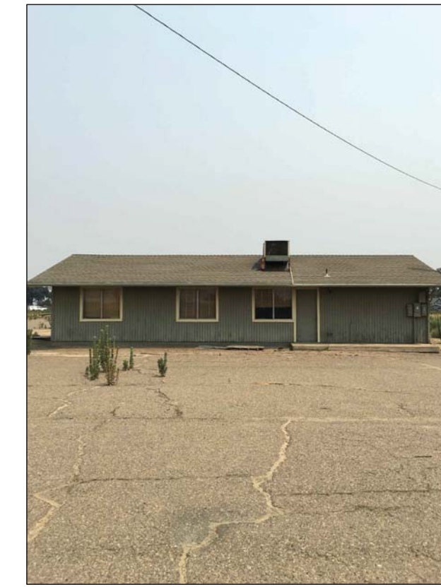
Existing Office - West
