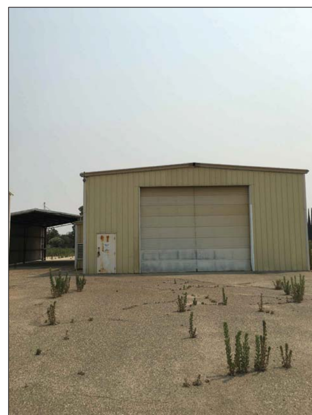
Existing Storage - North
