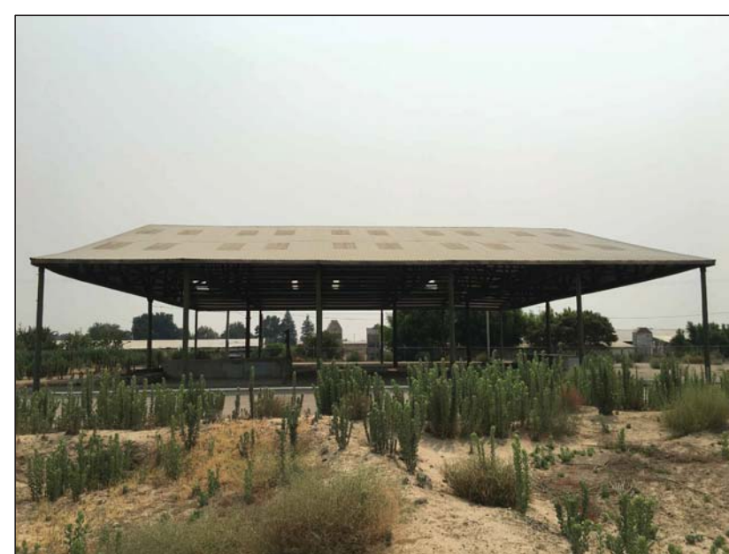
Existing Storage Pole Barn - North
