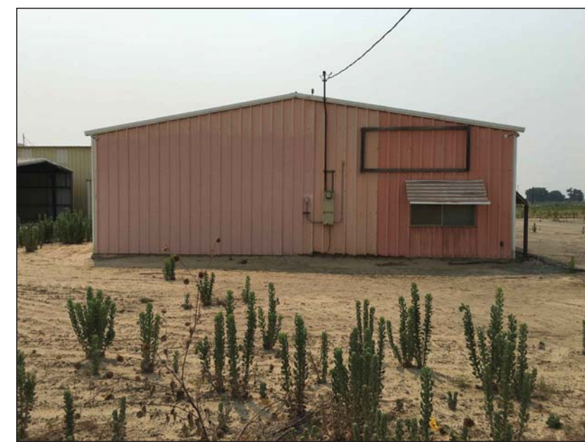
Existing Shop - East
