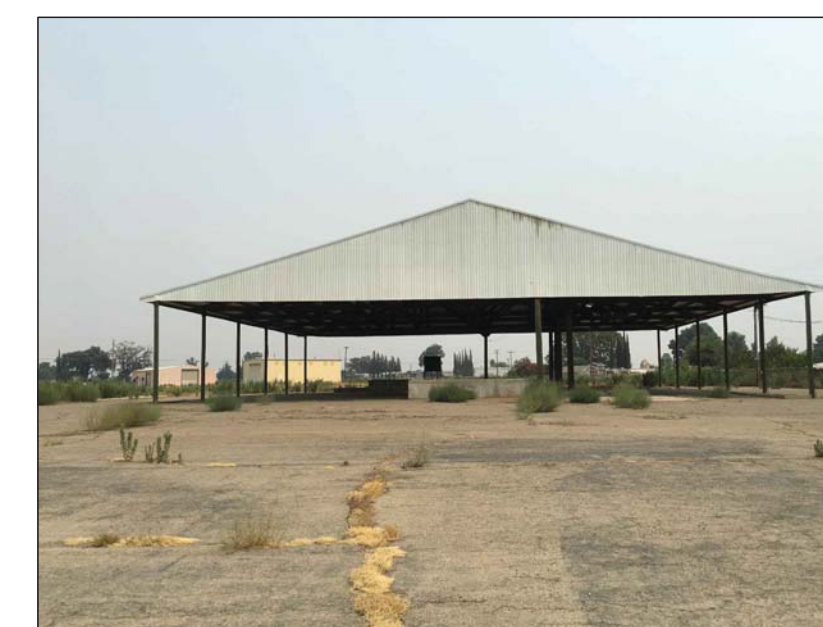
Existing Storage Pole Barn - West
