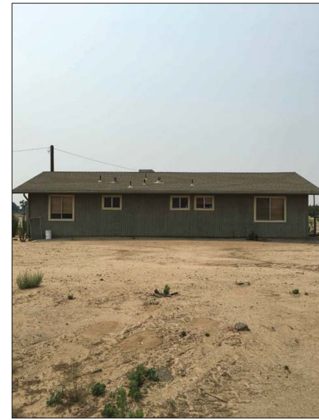
Existing Office - East
