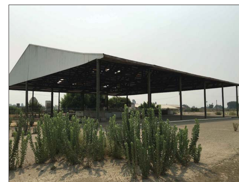
Existing Storage Pole Barn - South
