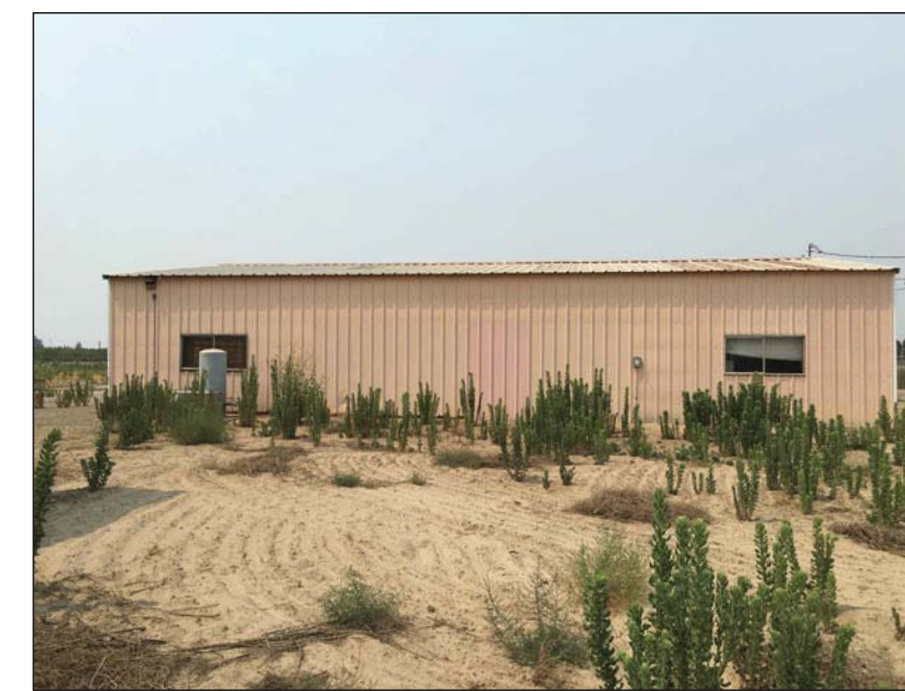
Existing Shop - South
