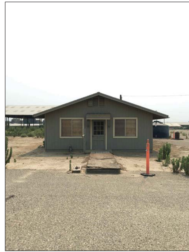
Existing Office - North
