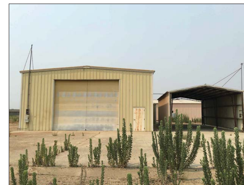
Existing Storage - South
