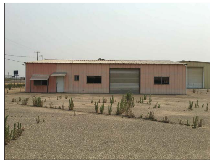
Existing Shop - North
