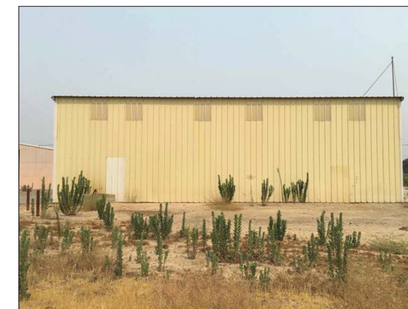
Existing Storage - West
