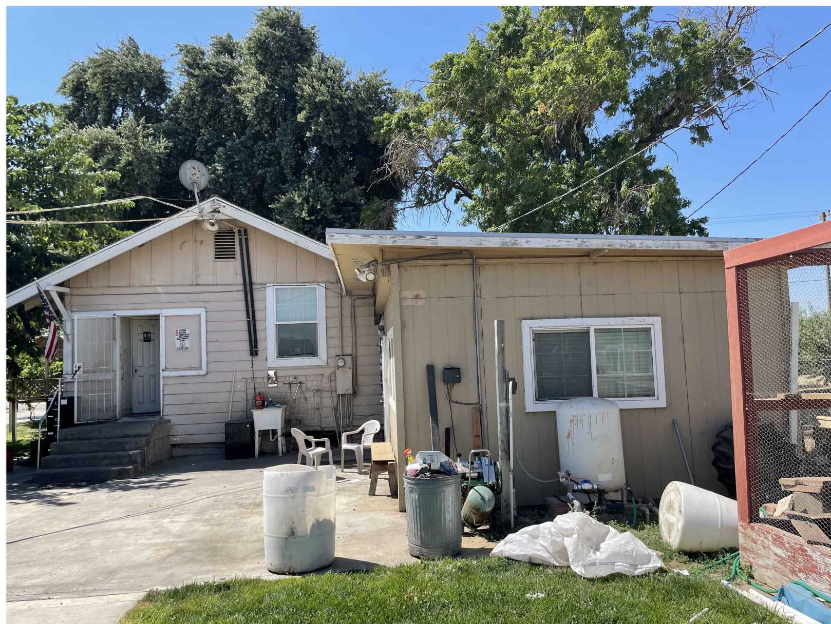
EXISTING OFFICE - NORTH
