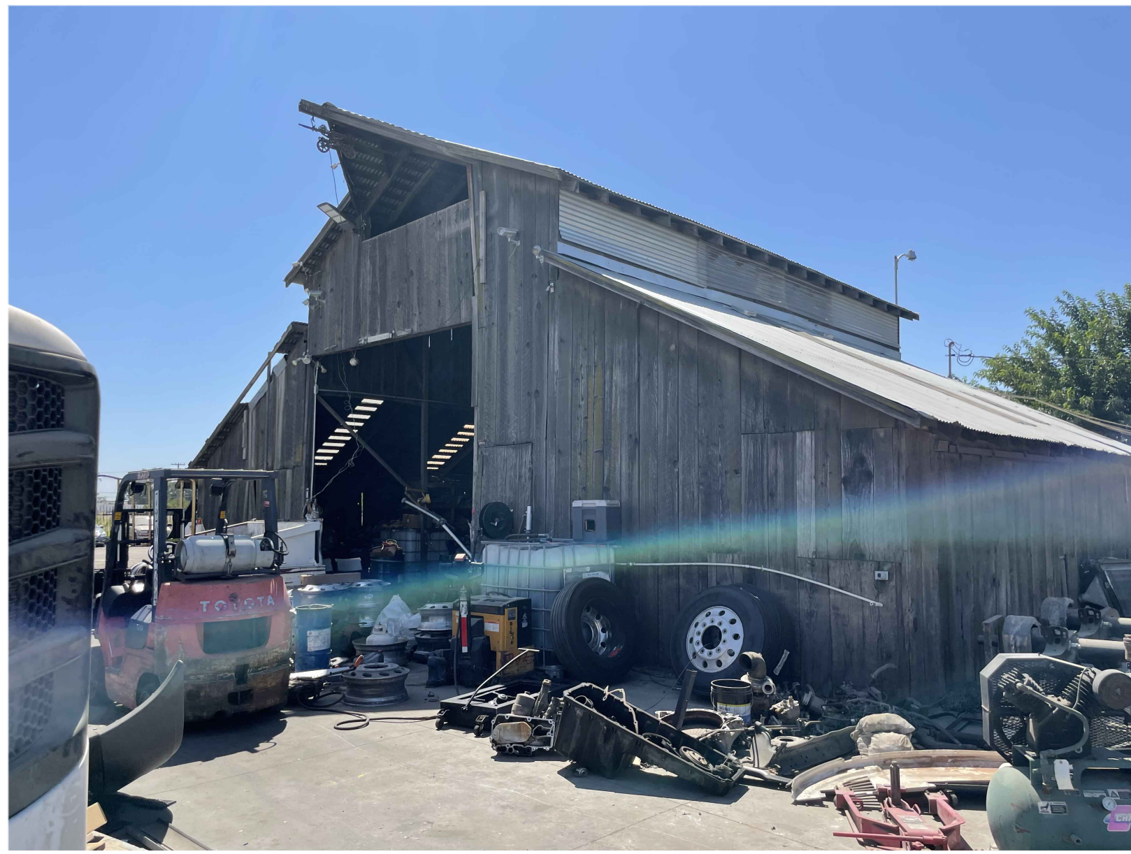
EXISTING SHOP - NORTH
