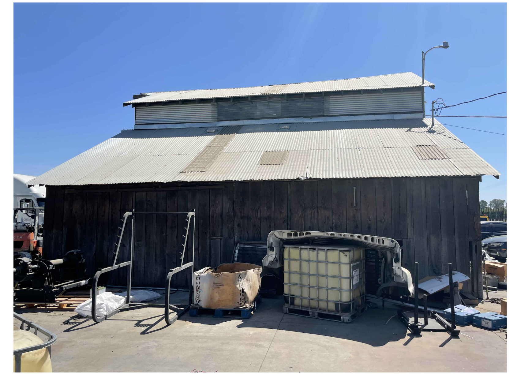
EXISTING SHOP - WEST
