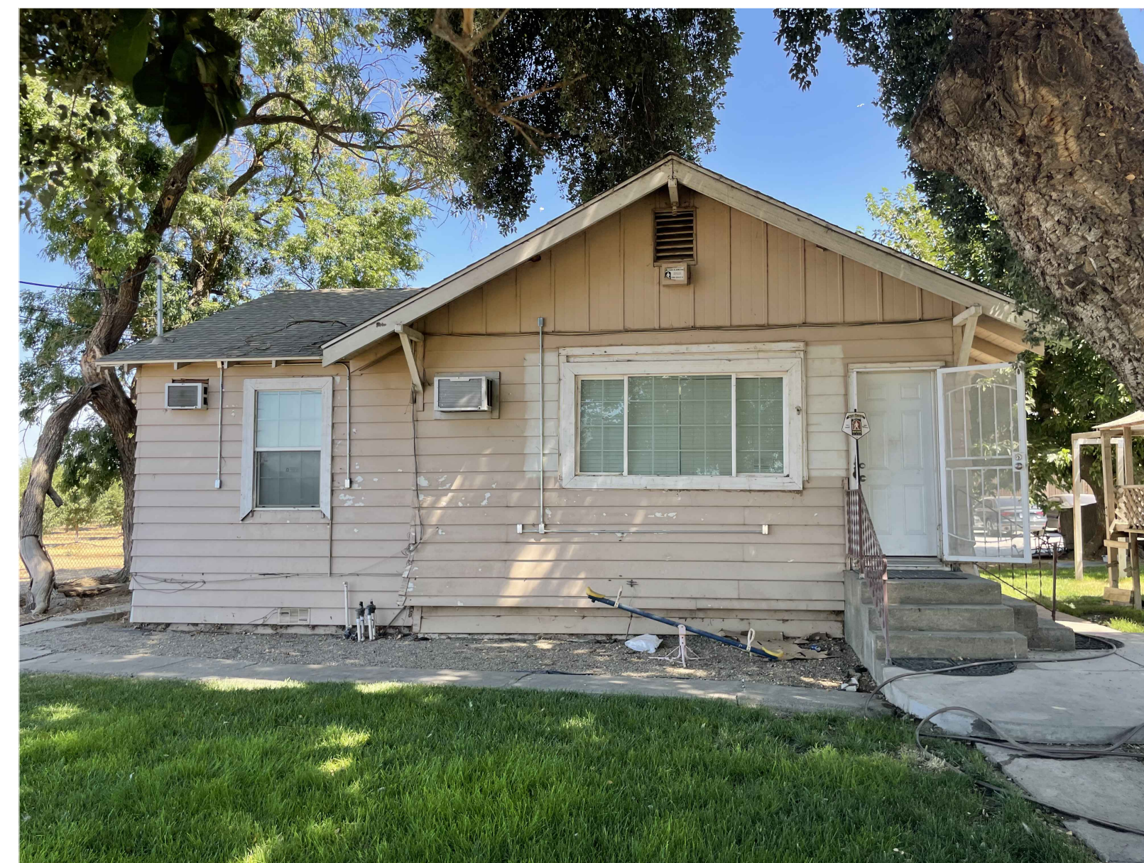
EXISTING OFFICE - SOUTH
