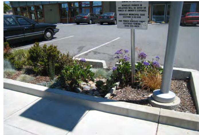
Stormwater bioretention area in parking area.
