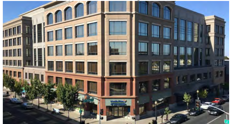
Photo 1- Tenth Street Place
