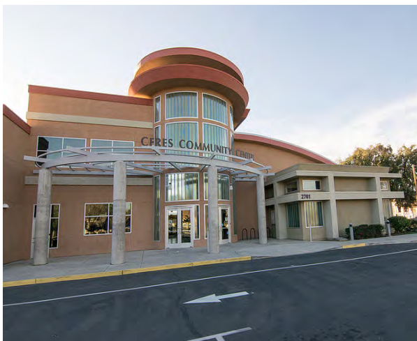
Photo 11 - Ceres Community Center
