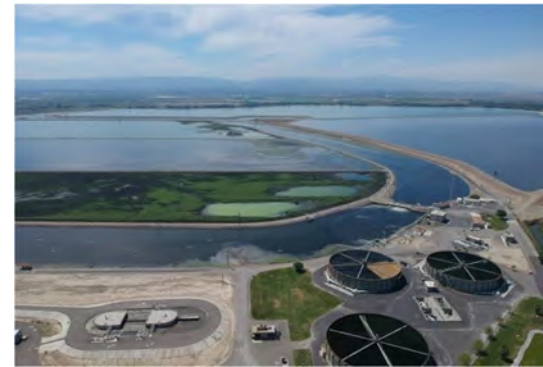
Modesto's Jennings Water Treatment Plant
