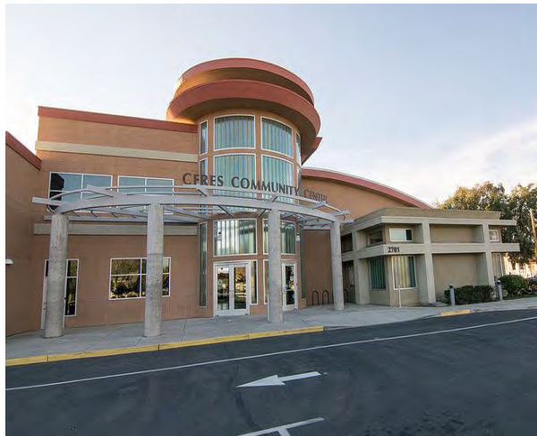
Photo 11 - Ceres Community Center
