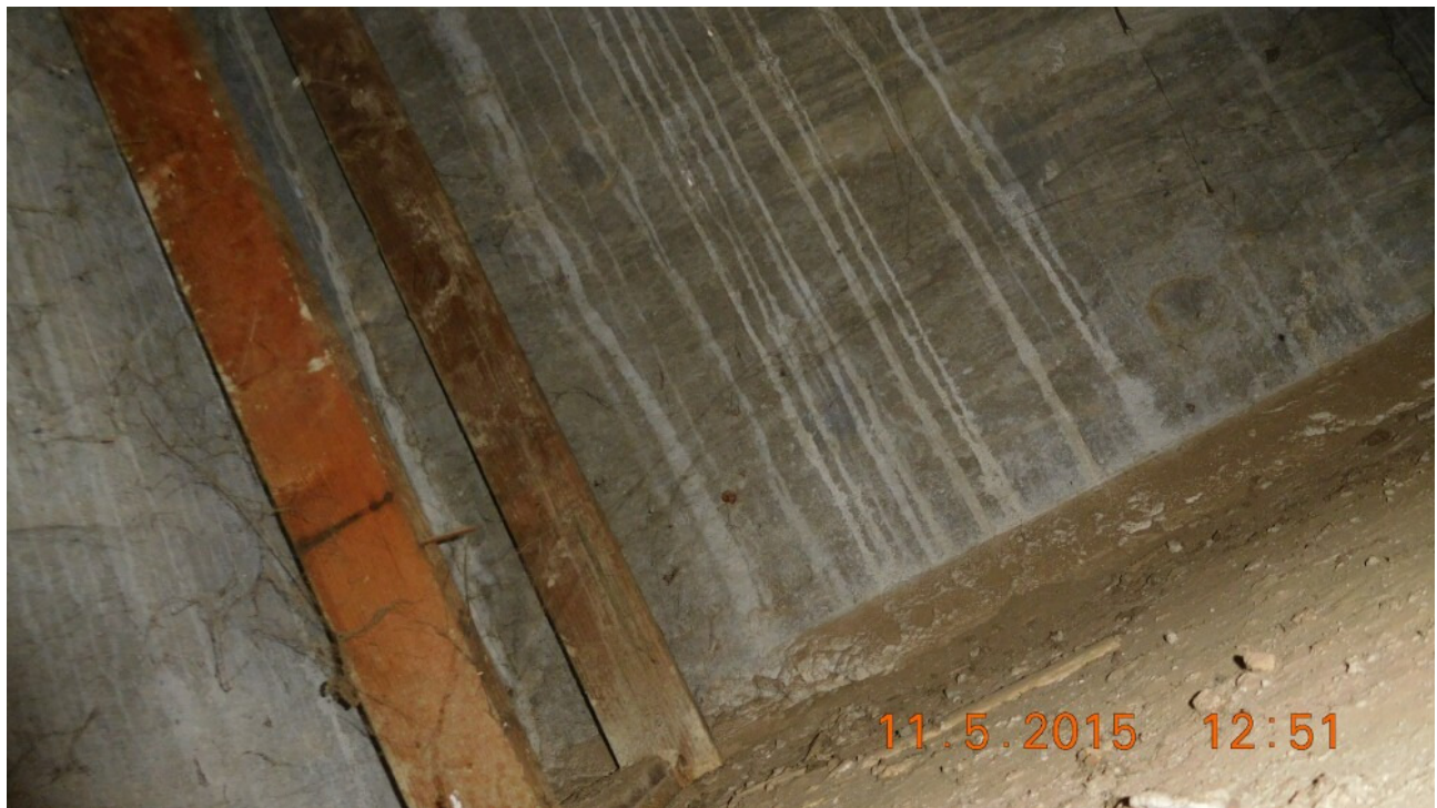
Figure 10. Interior of another girder cell.
