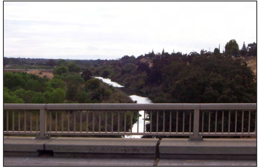
View west of the Tuolumne River from the Hickman Road Bridge.
