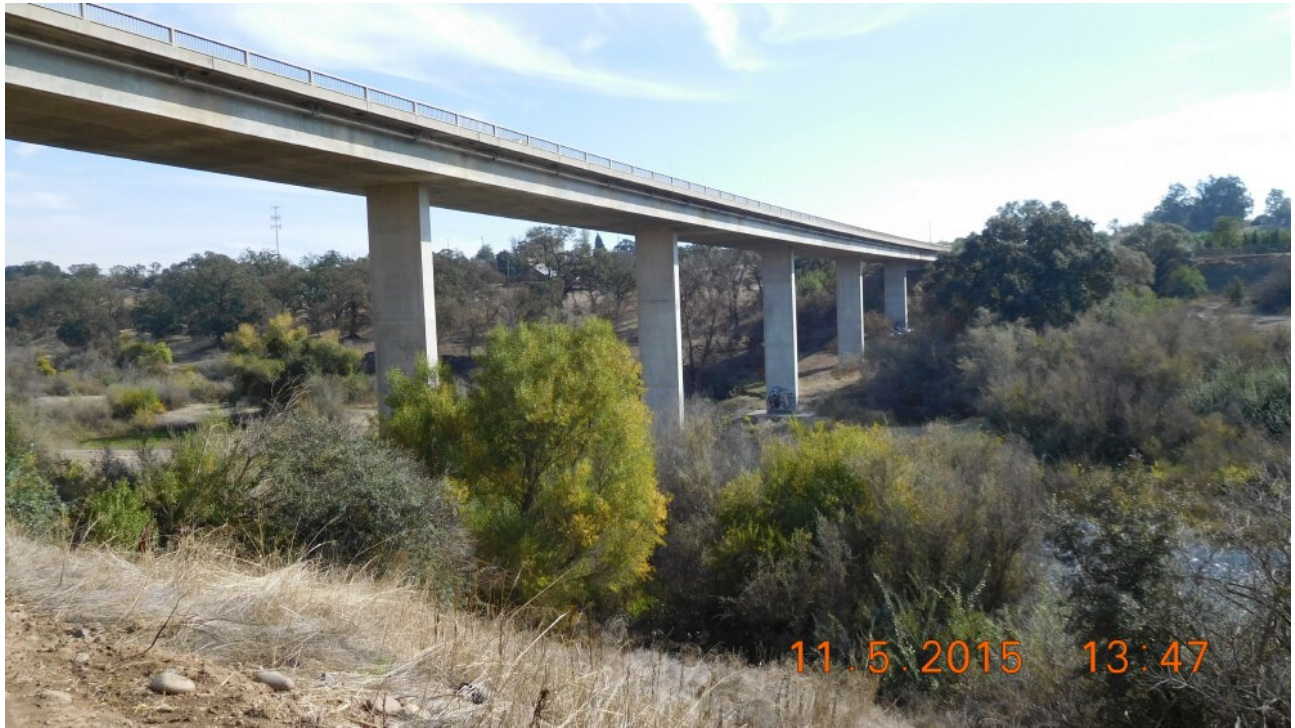
Figure 1. Hickman Road Bridge looking from north.
