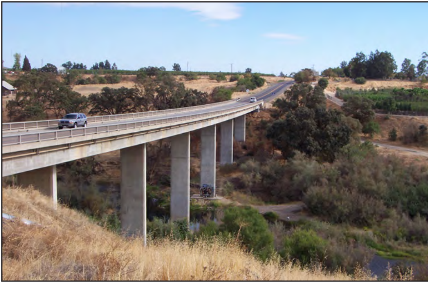
View northwest of the Hickman Road Bridge over the Tuolumne River.
