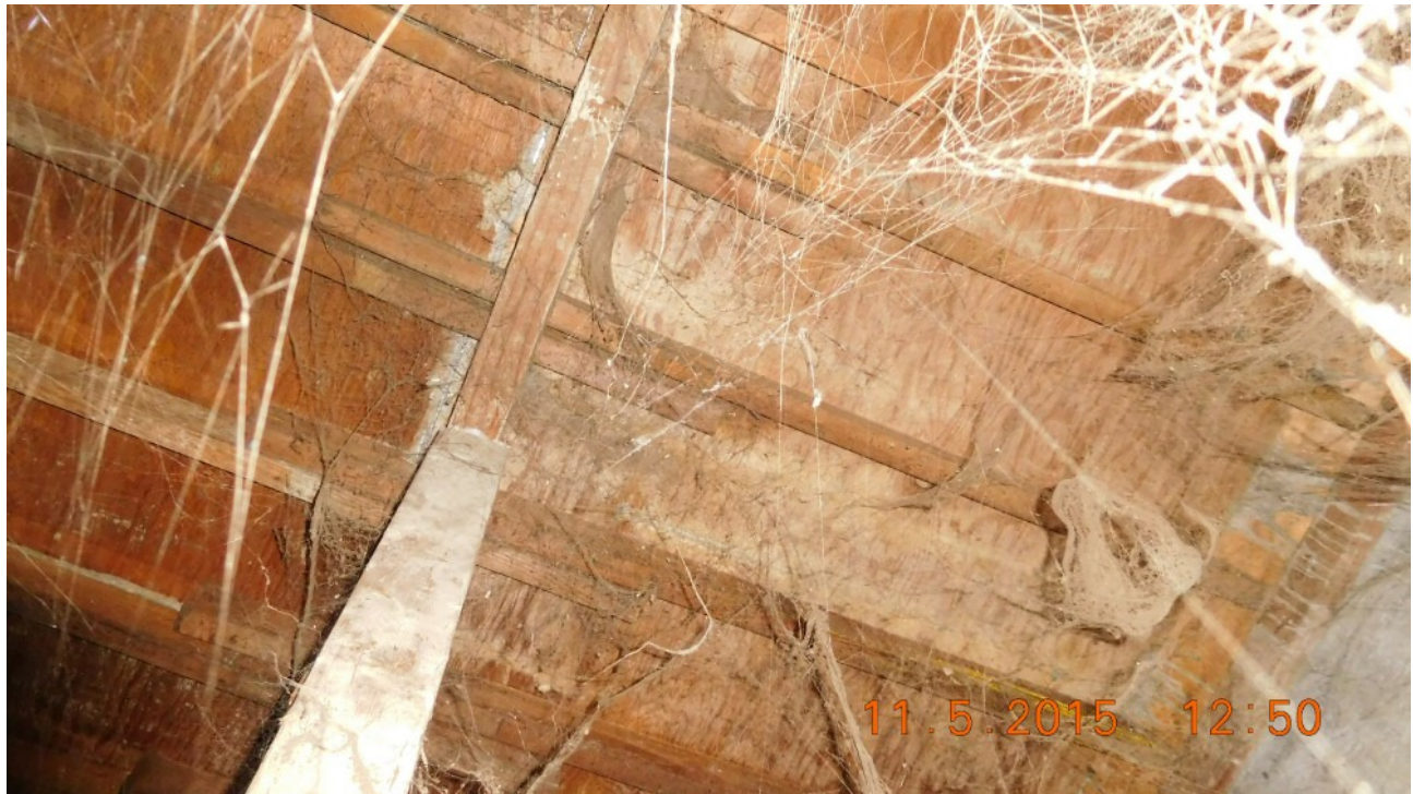
Figure 9. Interior of interior of one girder cell.
