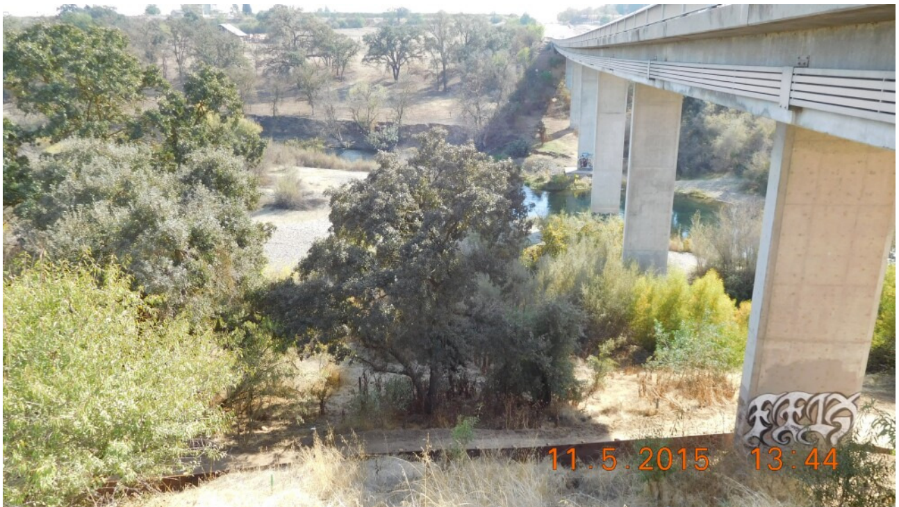
Figure 6. Hickman Road Bridge viewed from northeast abutment.
