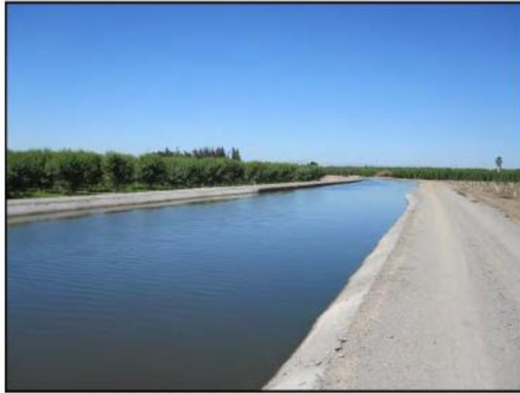
Photograph 7. View south of Lateral No. 6 Segment 2 with new gunite. Taken 5/27/14.
