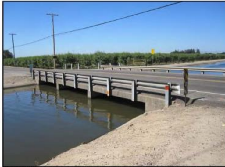
Photograph 8. View south of Feature I, Bridge 38C0228 carrying Coffee Road. Taken 5/27/14.
