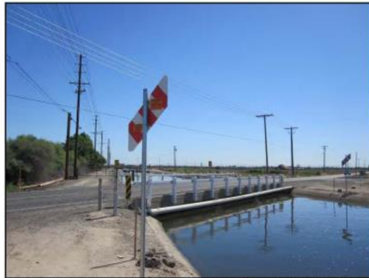
Photograph 4. View north of Feature G, Bridge 35C0113 on Claribel Road. Taken 5/27/14.
