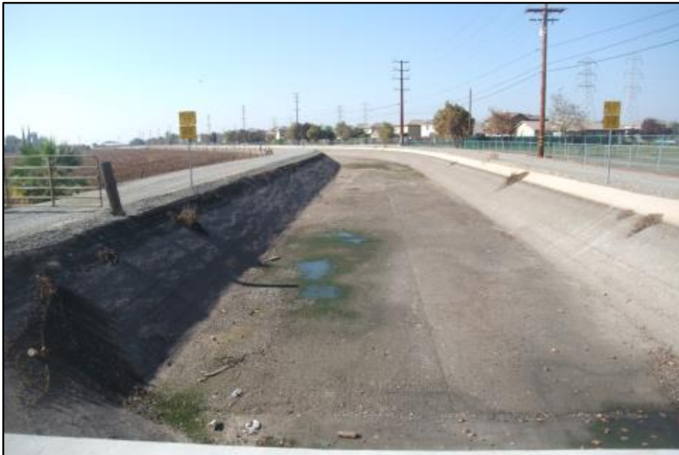
Figure 9. P-50-000075 MID Lateral No 6, view toward west.
