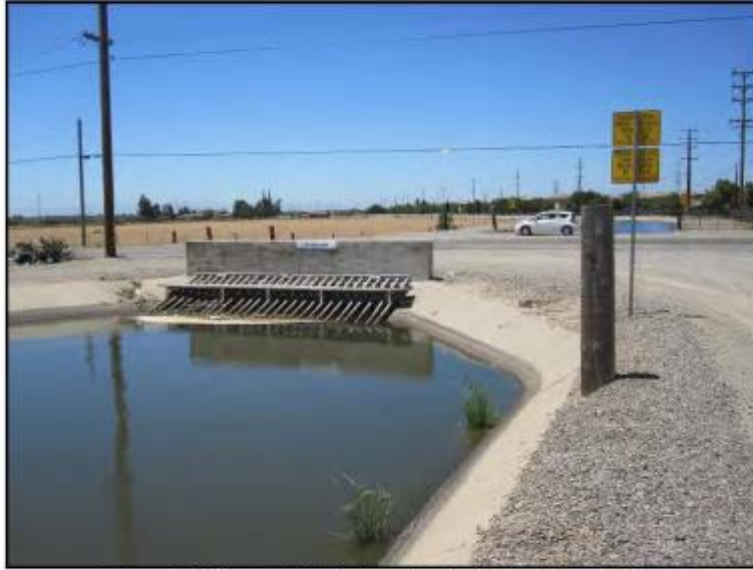
Photograph 5. View west of culvert carrying Roselle Road (Feature C).
