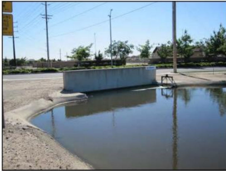
Photograph 3. View east of culvert under Oakdale Road (Feature D). Taken 5/27/14.
