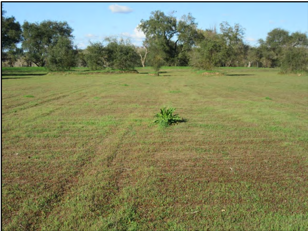
Recently graded area in the northwest part of the site, looking north; 01/19/18.
