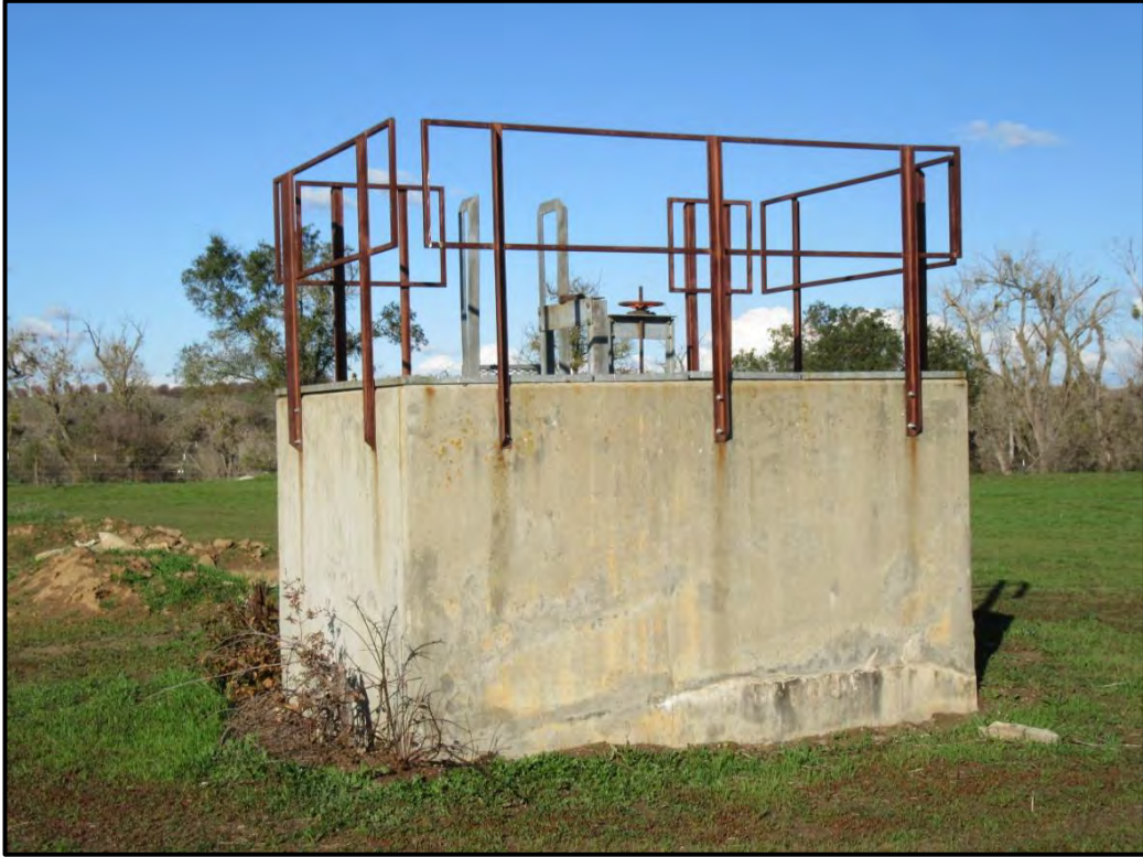
Irrigation structure located in the center of the site, looking northeast; 01/19/18. This structure is associated with an Oakdale Irrigation District pipeline through the site.
