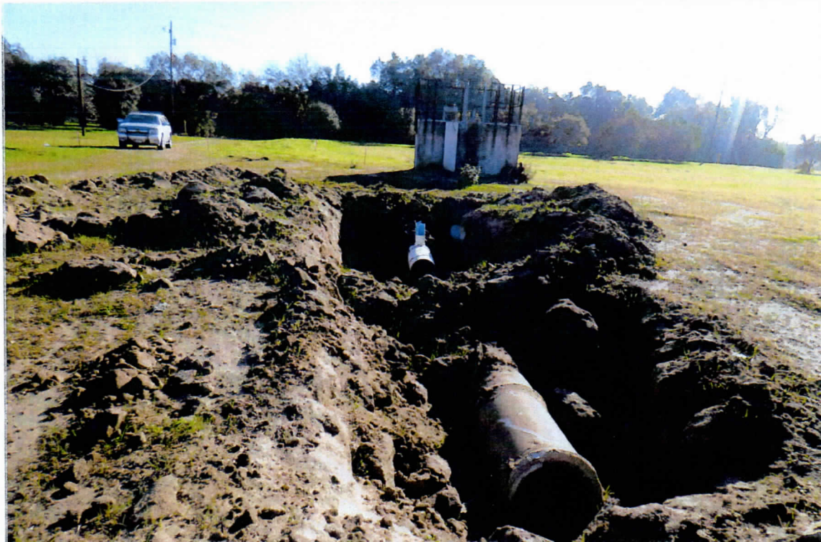
Figure 4: View south showing disused Gray Pipeline exposed by recent excavation.
