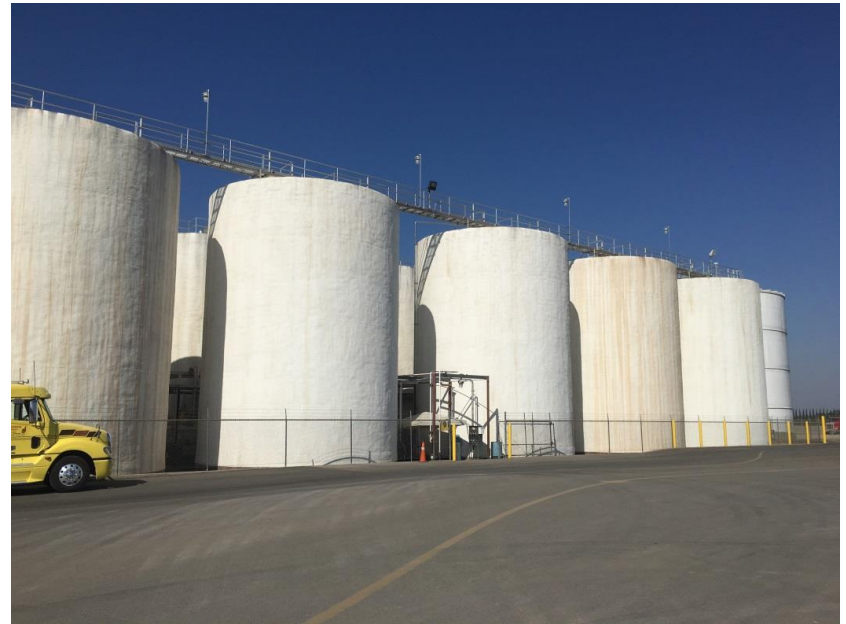
SOUTHEAST PORTION OF SITE EXISTING WINE TANKS
