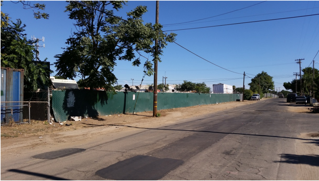
Looking northwest from Bystrum Road, south of Sousa Road. Required fencing and landscaping not installed.
