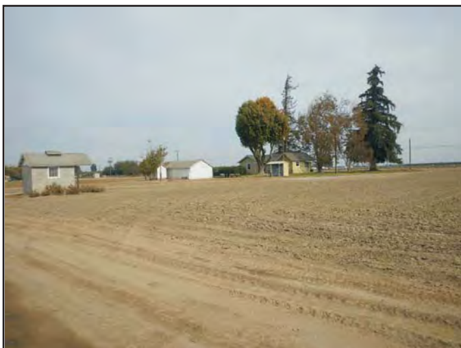
Photo 3: Dwelling and outbuildings in northern portion of operations area.
