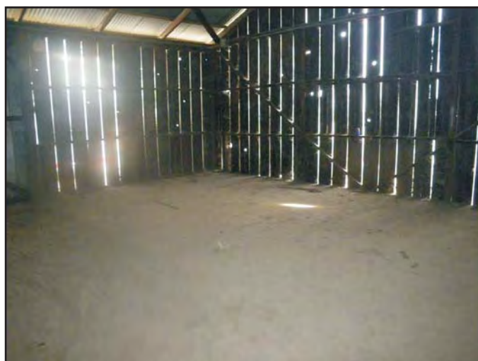
Photo 9: Eastern portion of barn/ packing shed with dirt floor.
