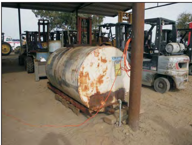
Photo 15: Waste oil tank in pole barn.
