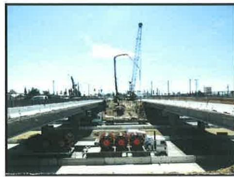
Stage 3: Abutment 1 Start Piles
