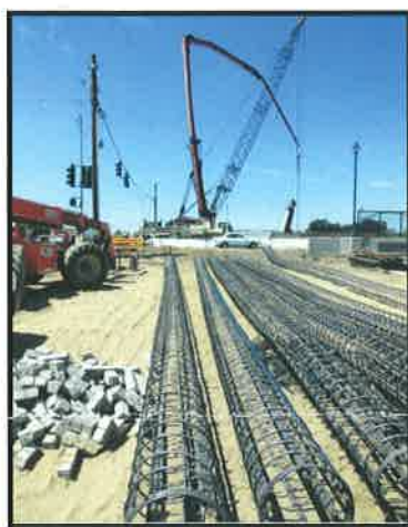
Stage 3: Start of Abutment 1 Construction and Pile Foundation
