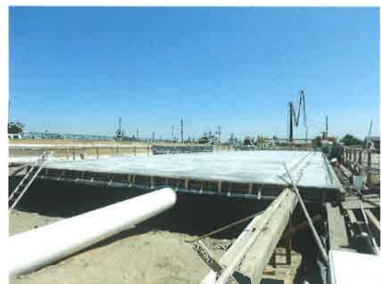
Stage 2: Bridge Completed Deck Pour
