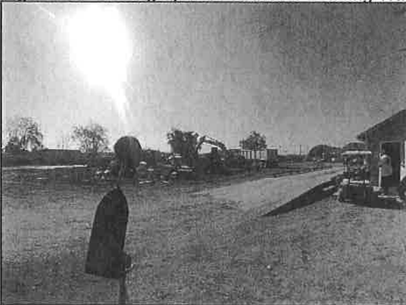
Figure 5c – Photograph of Excavator Loading Transfer Truck
