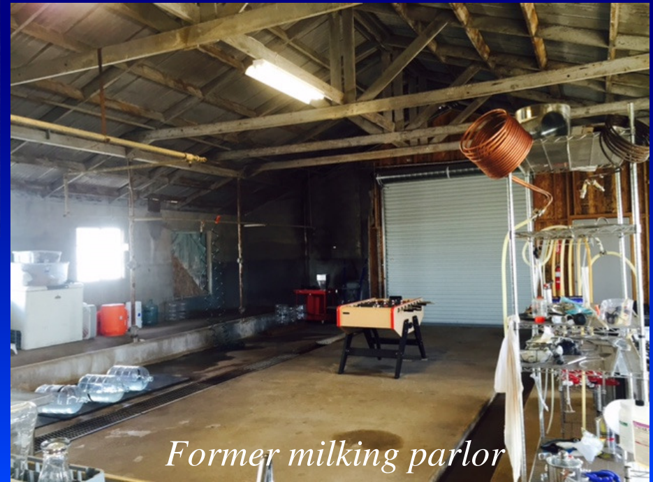
Former milking parlor
