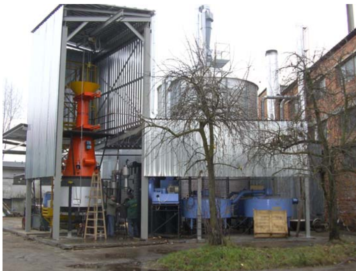
Figure 2 – The P250 biomass conversion chamber (red) and filtering system (blue)
