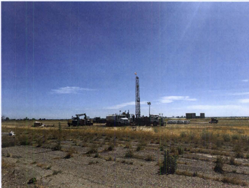
Figure 6 (below): Well Drilling Equipment by the runway.
