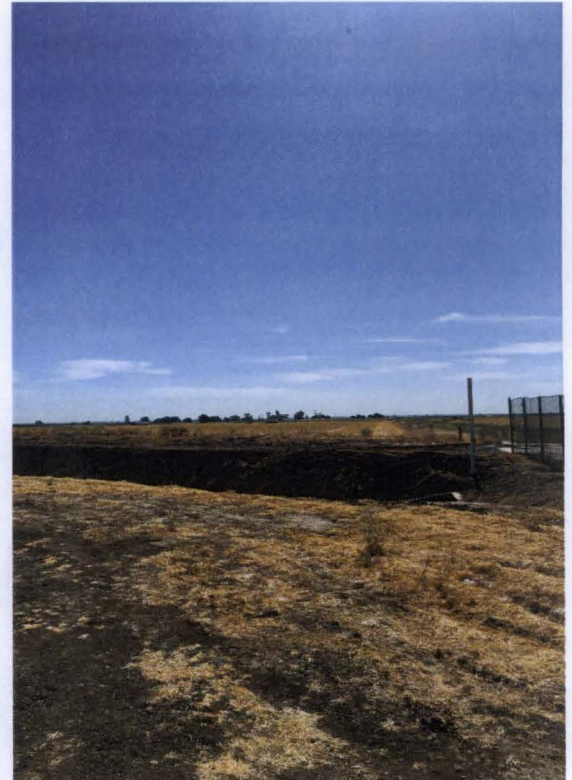
Figure 5 (right): Little Salado Creek Bank with Fenced Bridge.
