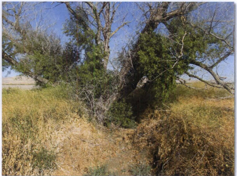
Figure 11: Large willow tree that is obstructing the culvert. No water present in the ditch.
