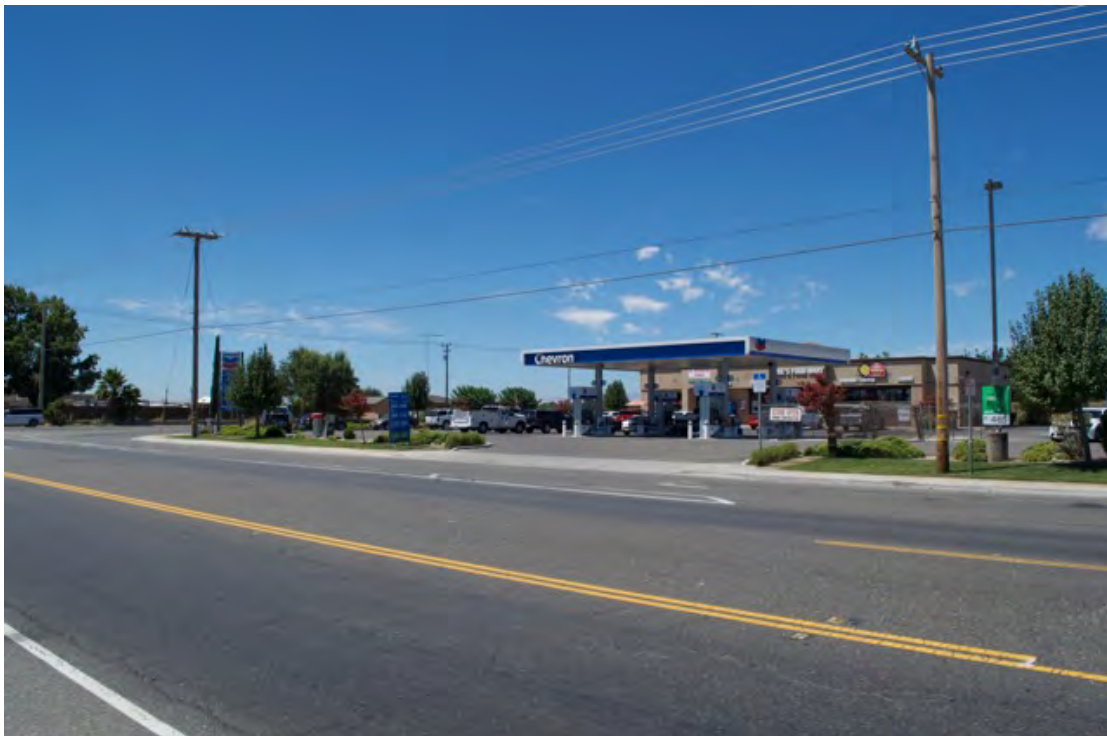
Photo 4 – Service station at northwest corner of project intersection, viewed west. USTs are adjacent to the right side of the canopy.
