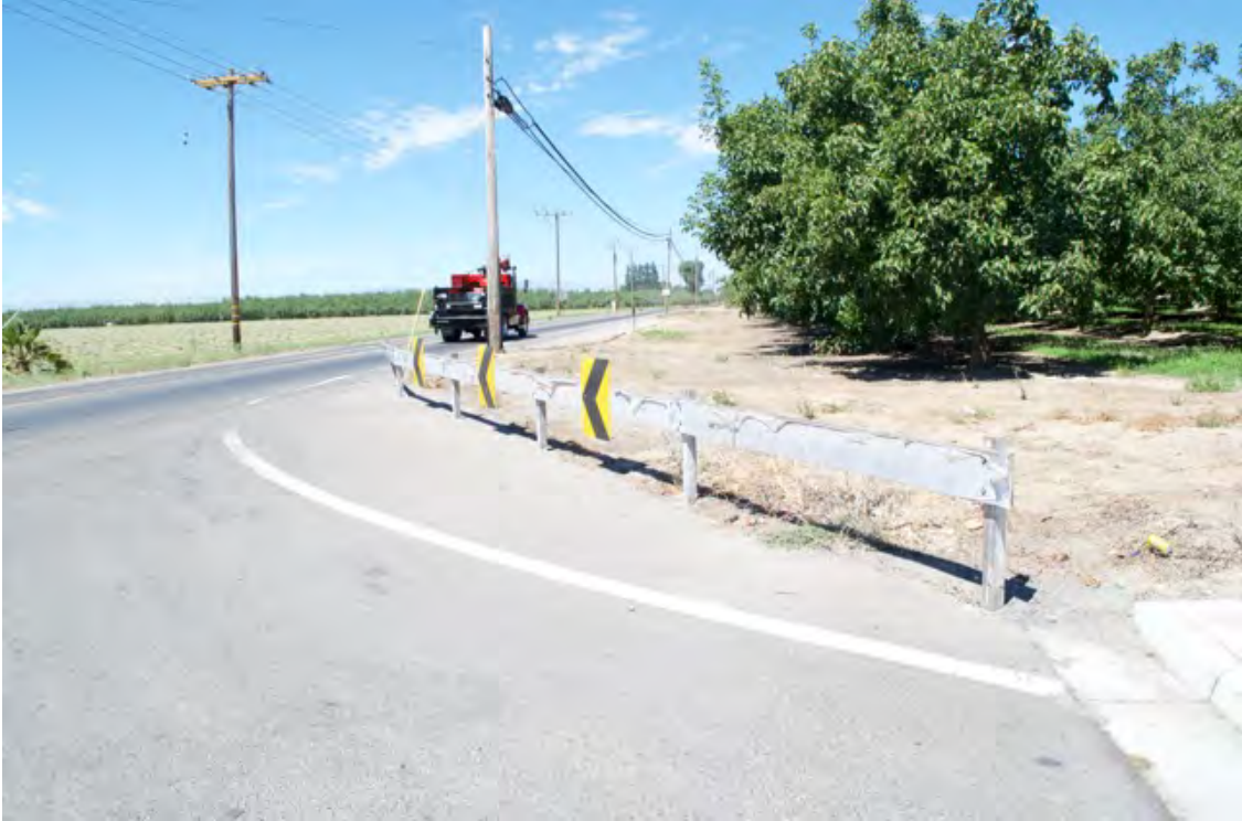
Photo 7 – Wooden guard rail on Grayson Road adjacent to service station property.
