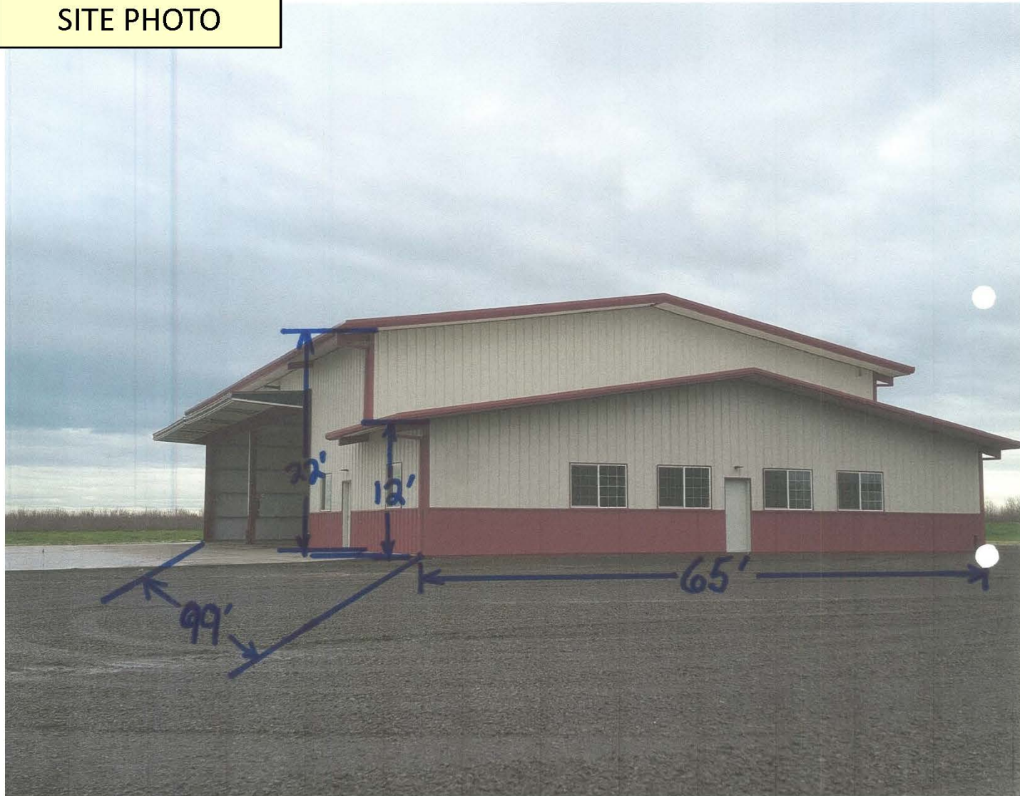
EXISTING AG STORAGE BUILDING
