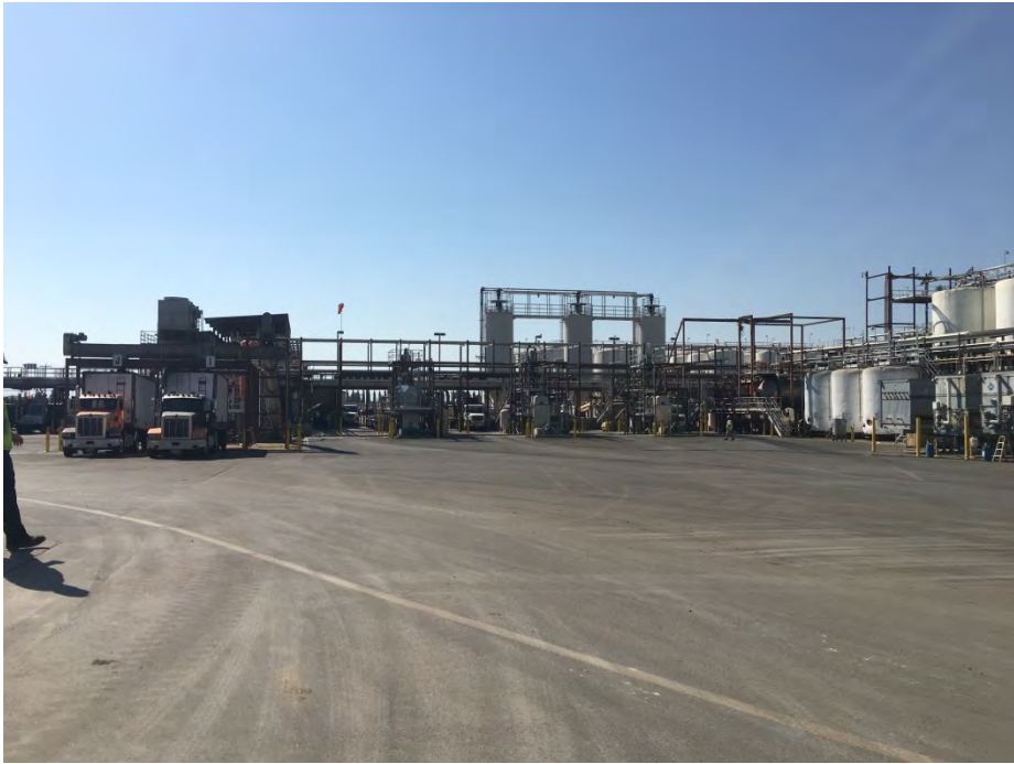
SOUTHEAST PORTION OF SITE EXISTING WINE TANKS & TRUCK DOCKS
