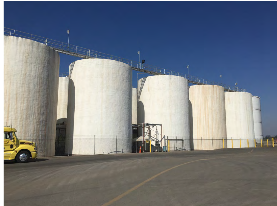
SOUTHEAST PORTION OF SITE EXISTING WINE TANKS
