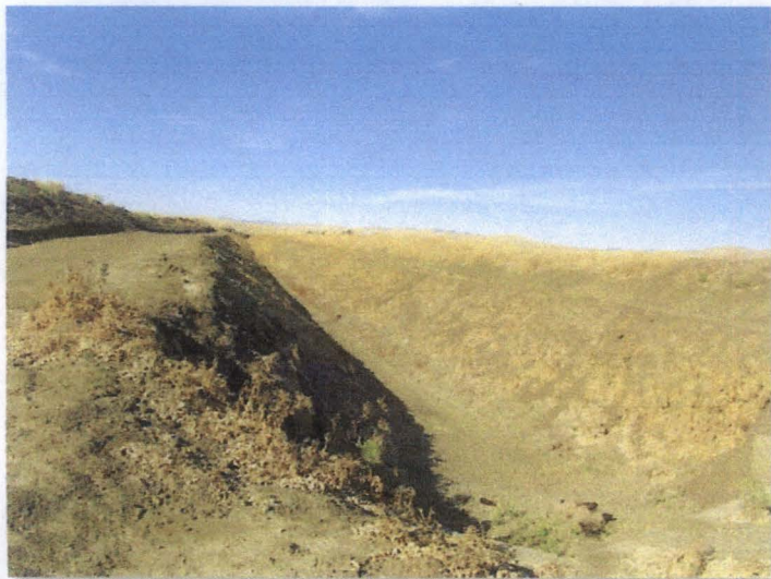
Figure 5 (below): Little Salado Creek is cleared of vegetation.
