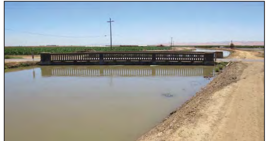
Looking at Shiells Road Bridge from the south.
