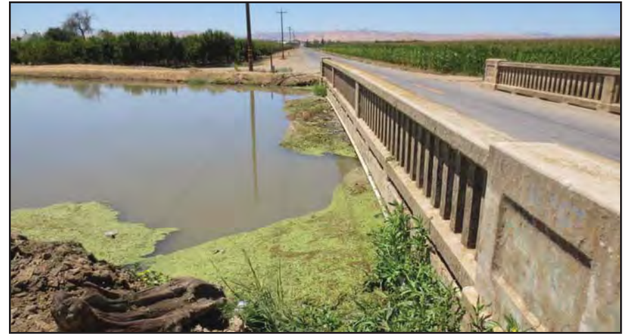
Looking at the Shiells Road Bridge from the east.
