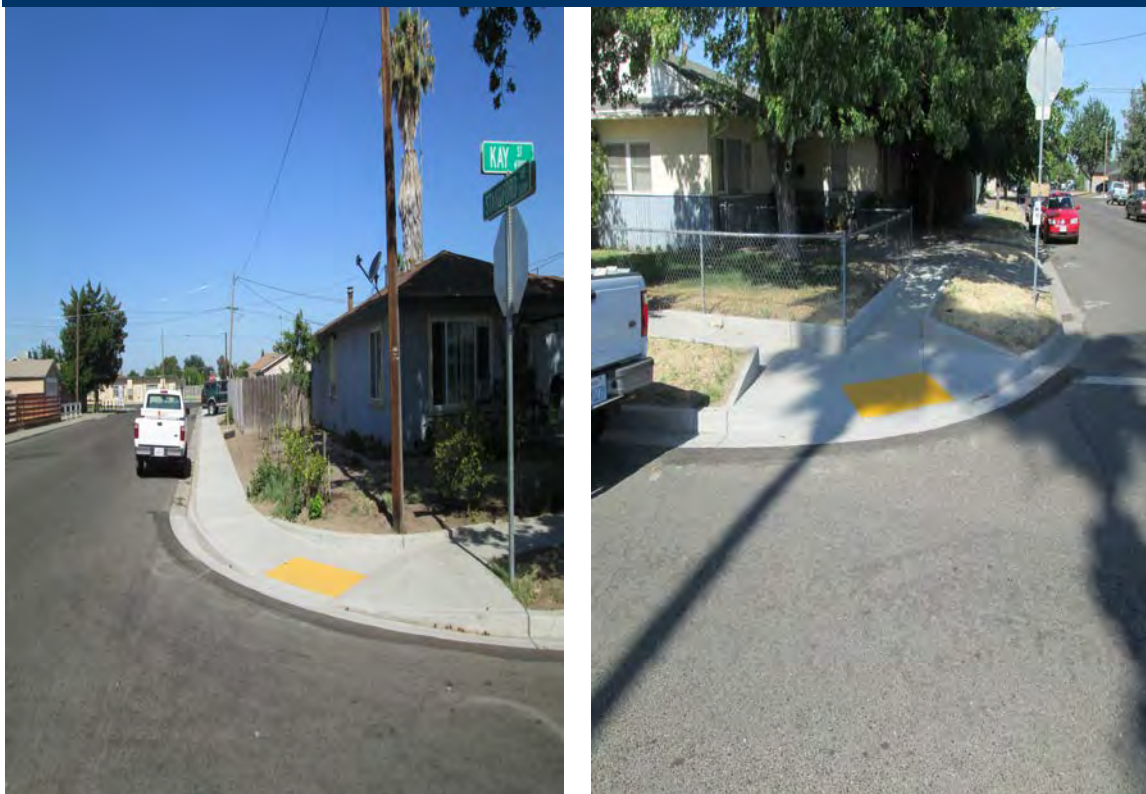
Photos reflect ADA ramp improvements within the project area.
