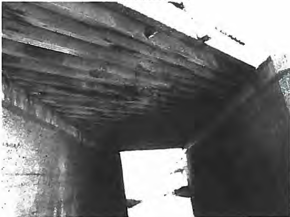
Photo No. 6 Underside of Span 2
