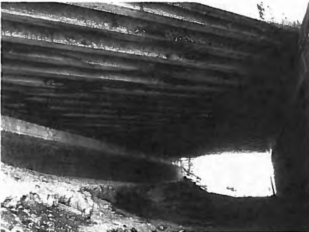
Photo No. 8 Underside of Span 4
