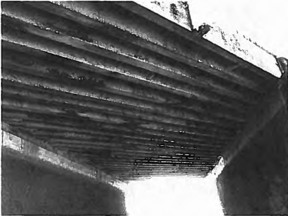
Photo No. 7 Underside of Span 3
