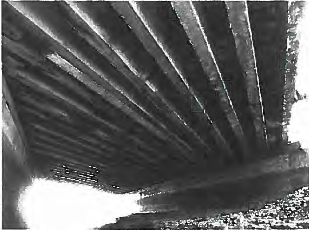
Photo No. 5 Underside of Span 1
