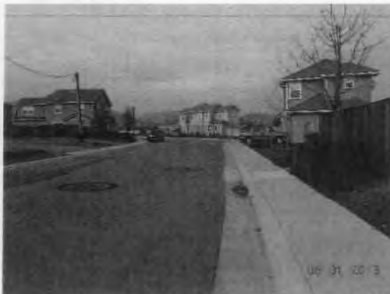
5 – Grapevine Drive (south end) looking north
