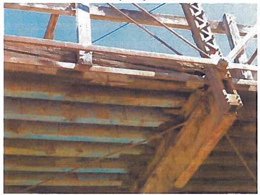
Photo No. 8 Damaged left exterior stringer near the second floorbeam
