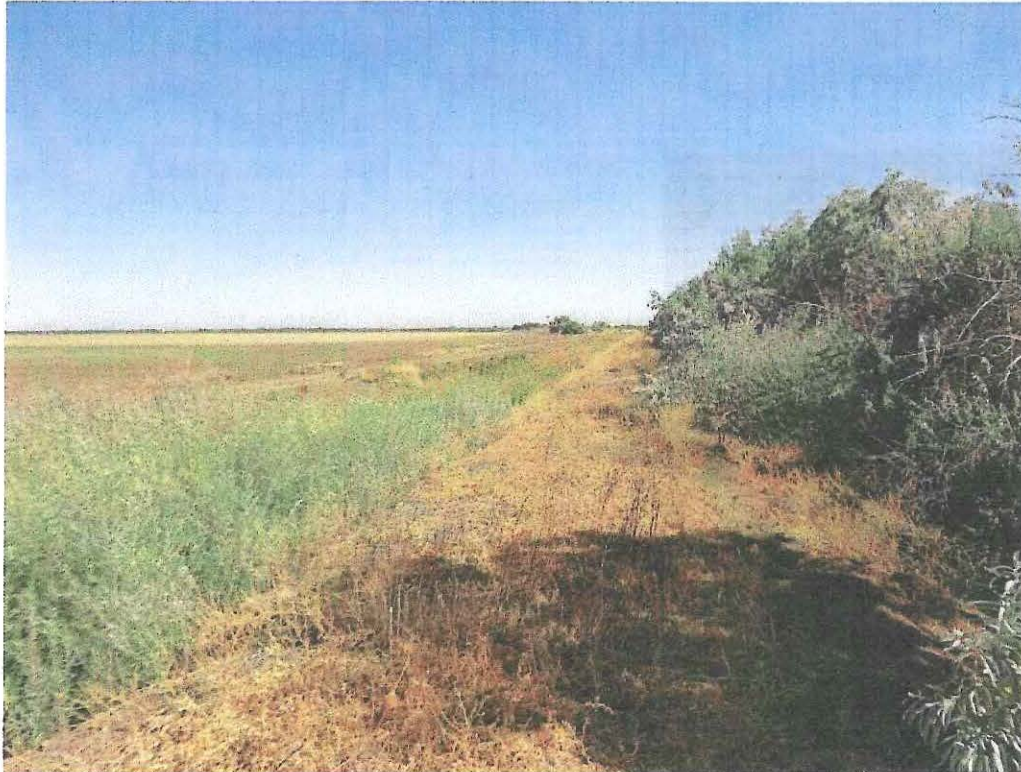
Figure 12. Marshall Drain, looking toward Marshall Road
