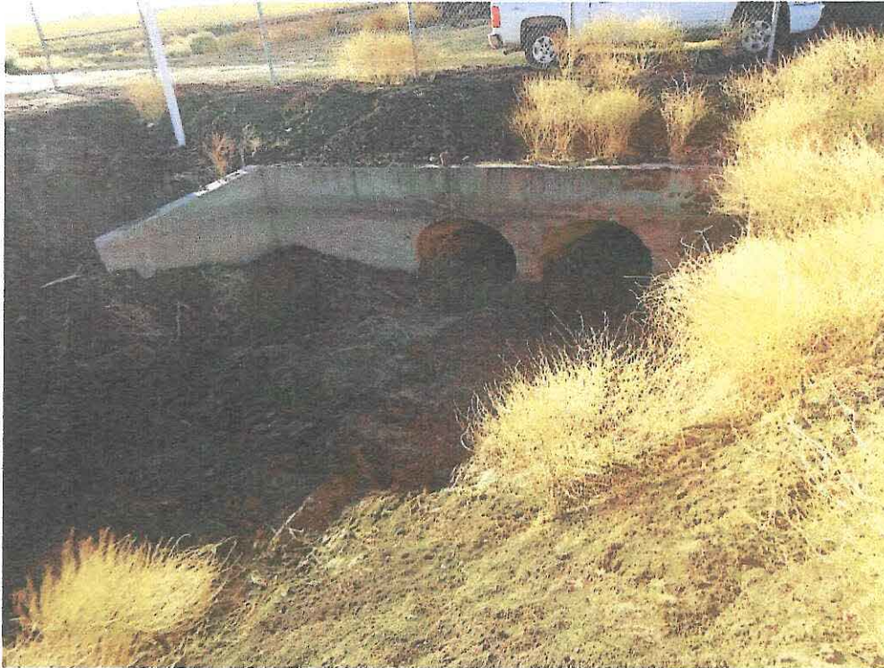
Figure 10. Drainage culvert, moderately congested (near Airstrip); significantly cleared out since 2013 monitoring
