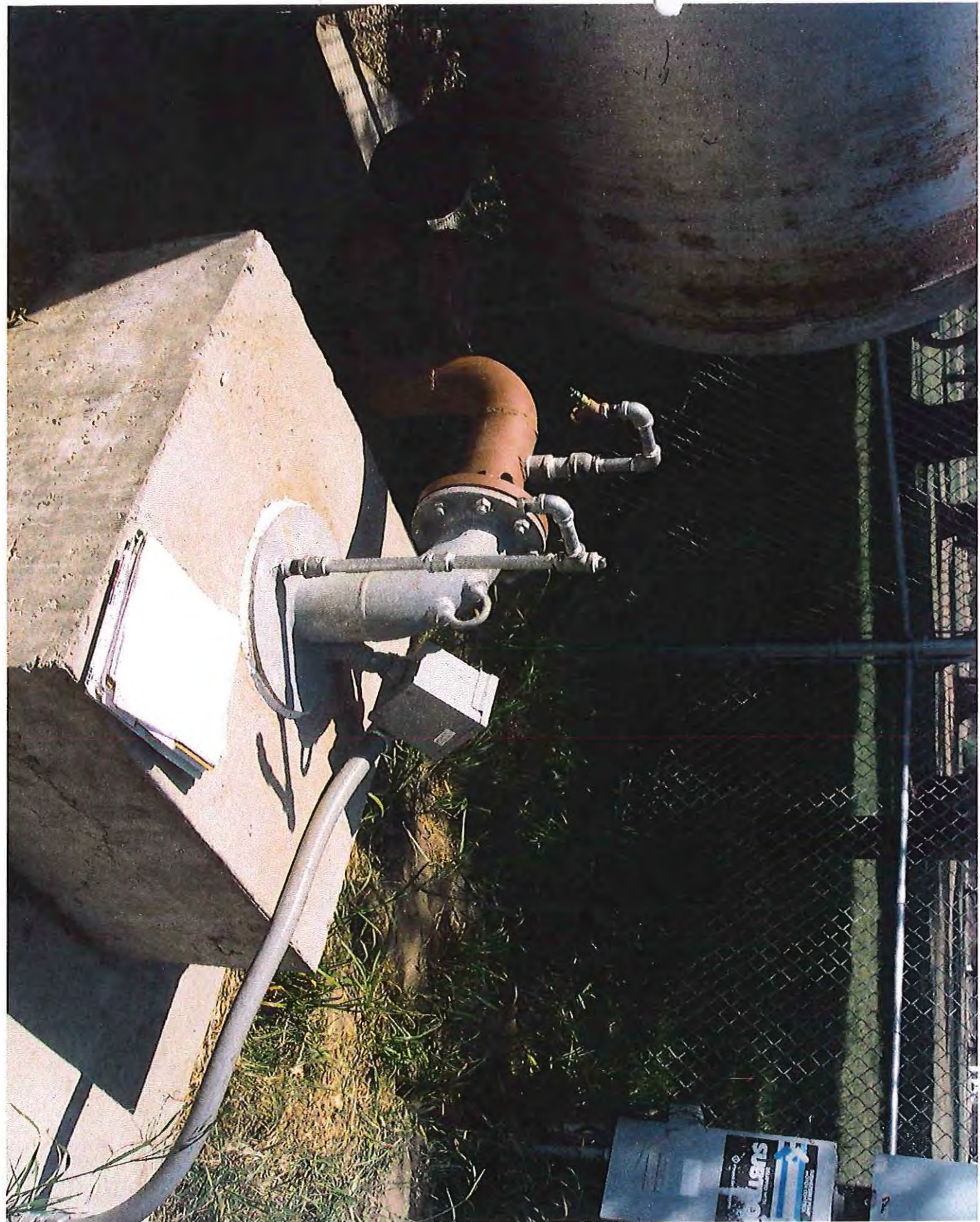
Samm-Co. Home Farm - Greystone Rd. Hwy 9129
