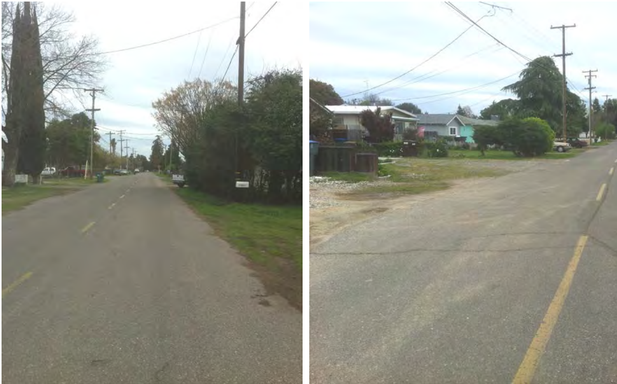
Photos reflect the La Gallina Avenue Infrastructure project area in need of curb, gutter, storm drain, and sidewalk.
