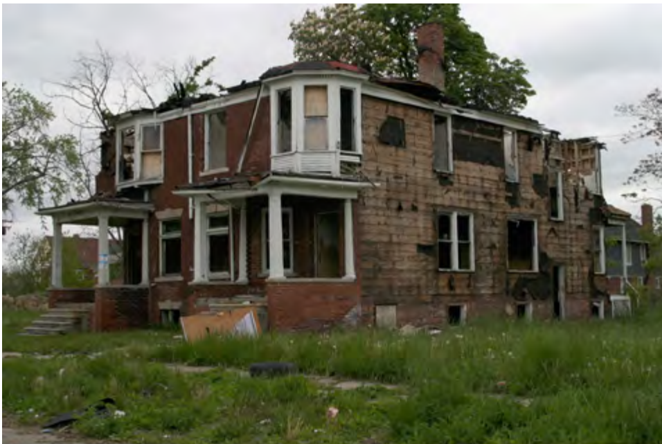
Abandoned house on Detroit's east side
