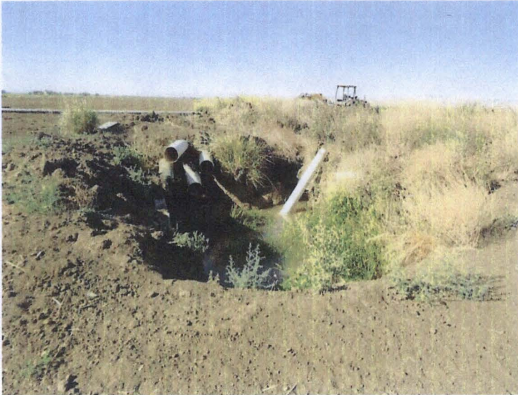
Figure 5. Irrigation drain, weeds
