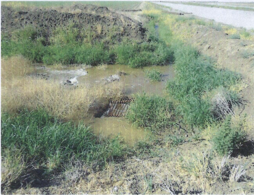
Figure 9. Irrigation drain, adjacent to field 10
