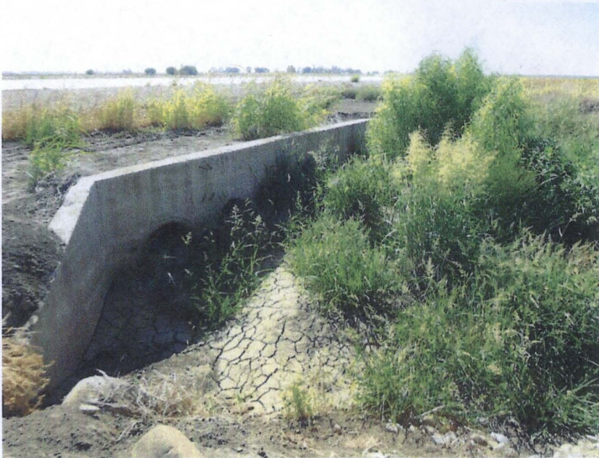
Figure 11. Drainage culvert, moderately congested (near Airstrip)
