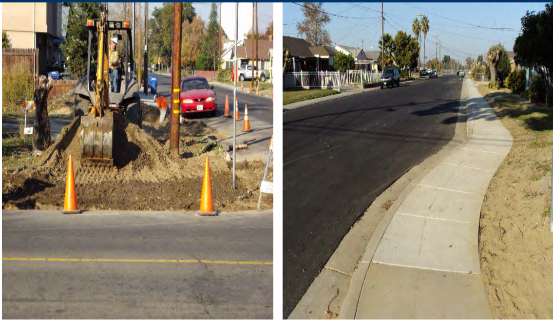
Photos reflect before and after work in downtown residential streets lacking curb, gutter, storm drain, sidewalks, and ADA ramps in Ceres.
