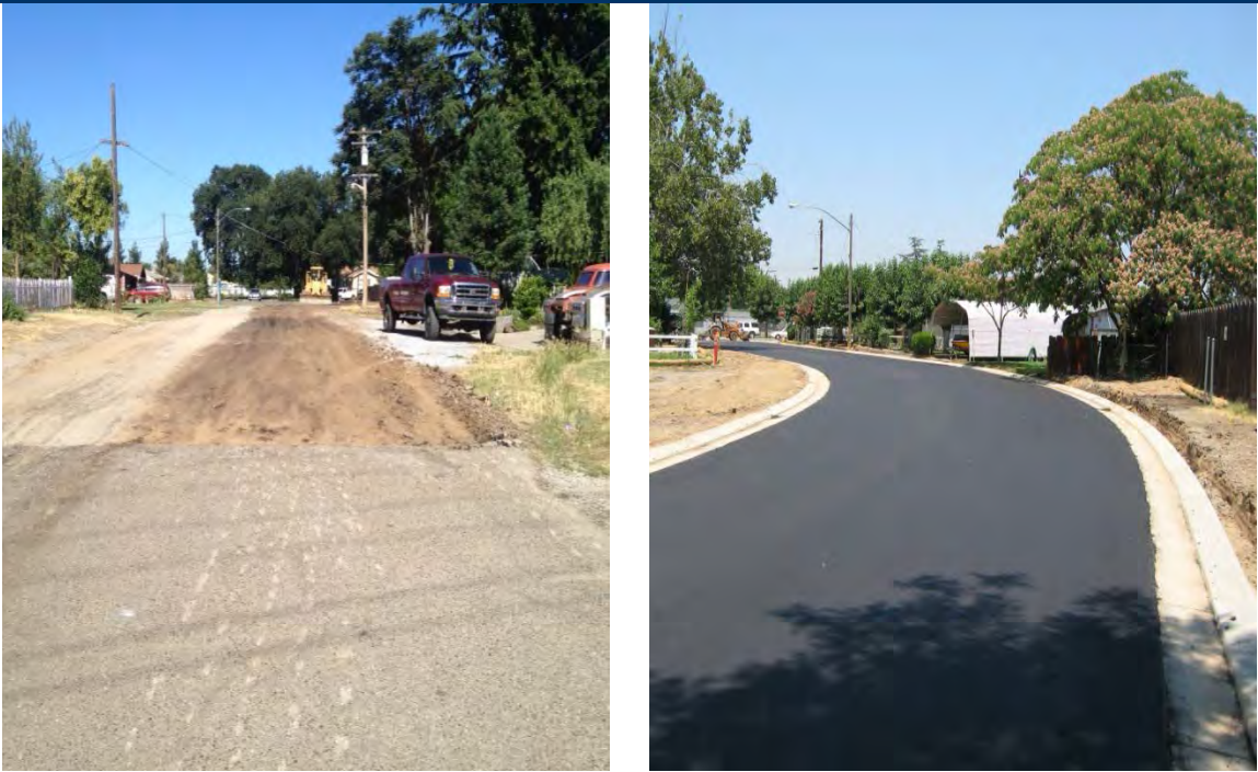
Photos reflect before and after the infrastructure improvements along Covey Street
