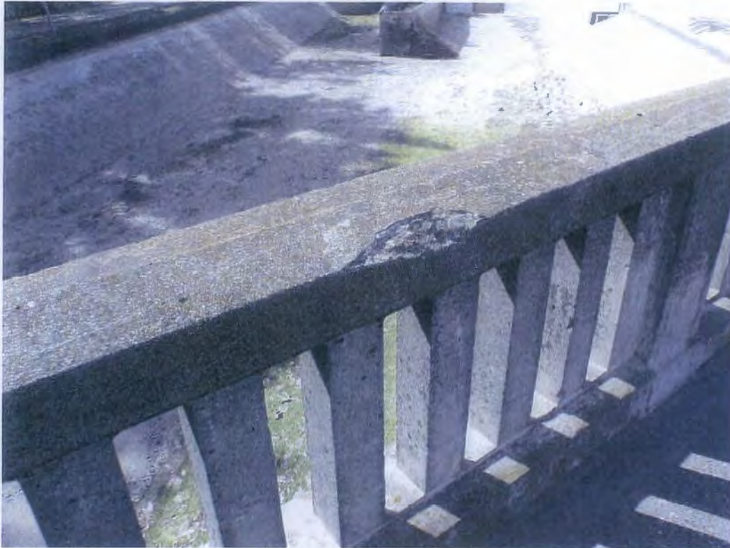
Photo No. 3 Right concrete rail
