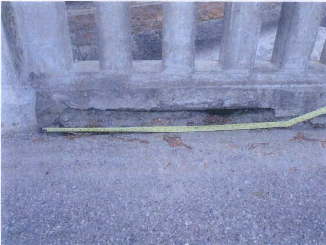
Photo No. 4 Right concrete rail near Abutment 5
