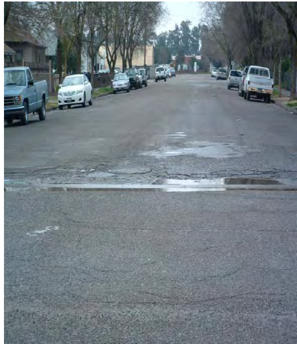
Photos reflect the Fifth Street project area in need of curb, gutter, storm drain, sidewalk, ADA ramps repair or installation and incidental street repaving. (Work to include underground water line replacement).
