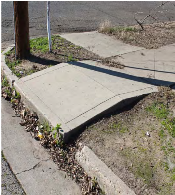
Photos reflect the Fifth Street project area in need of curb, gutter, storm drain, sidewalk, ADA ramps repair or installation and incidental street repaving. (Work to include underground water line replacement).
