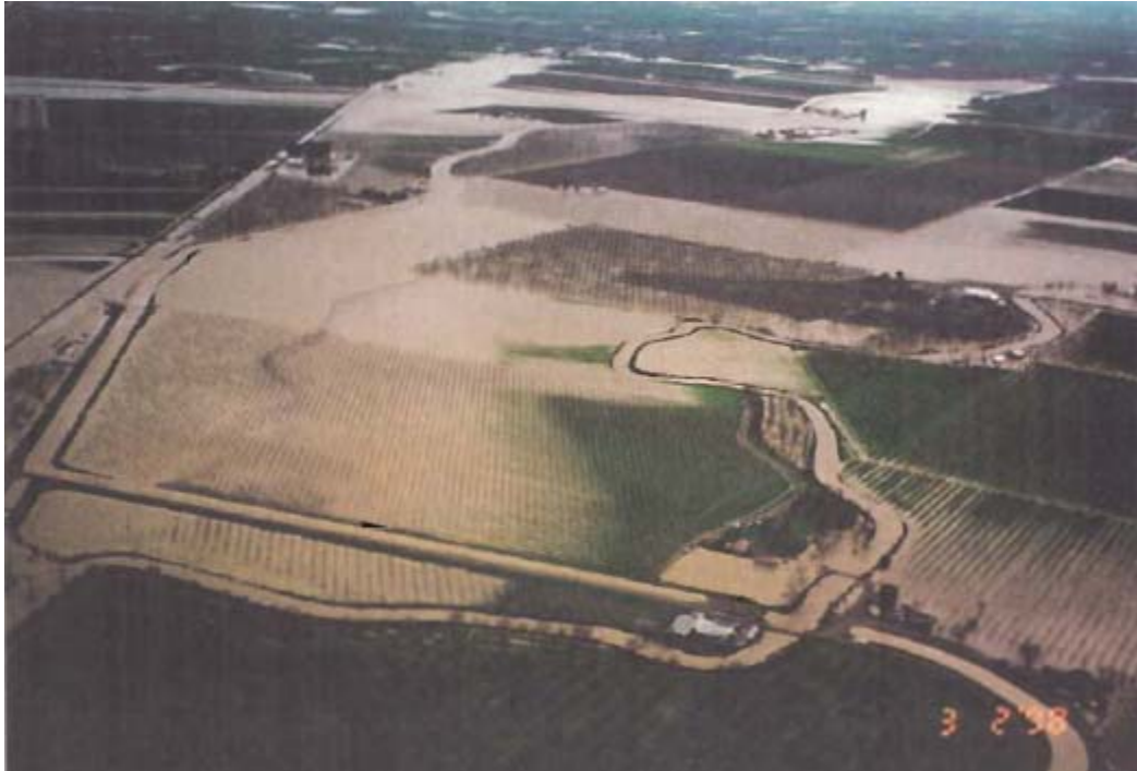
Figure 2-6: February 1998 Flooding from Orestimba Creek in the vicinity of the CCID Main Canal Siphon
