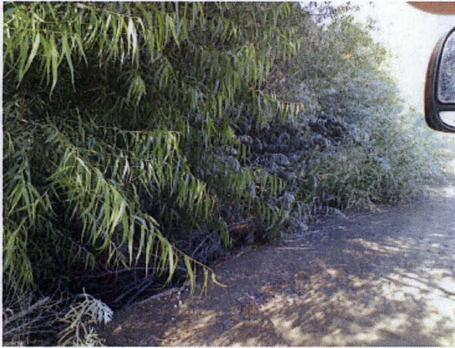
Figure 13. Marshall Drain, severely congested with vegetation and debris between field 2 and Wildlife Area
