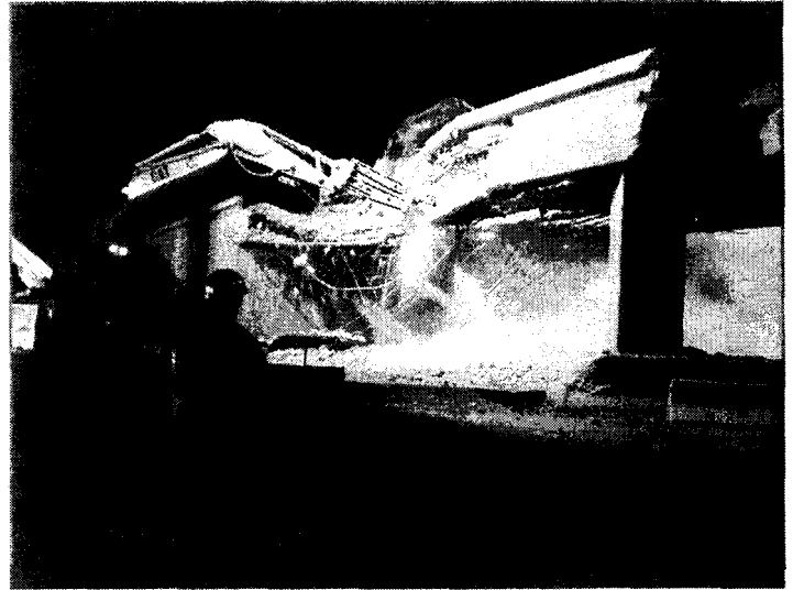
Jack Tone Road Bridge Demolition over SR 99
