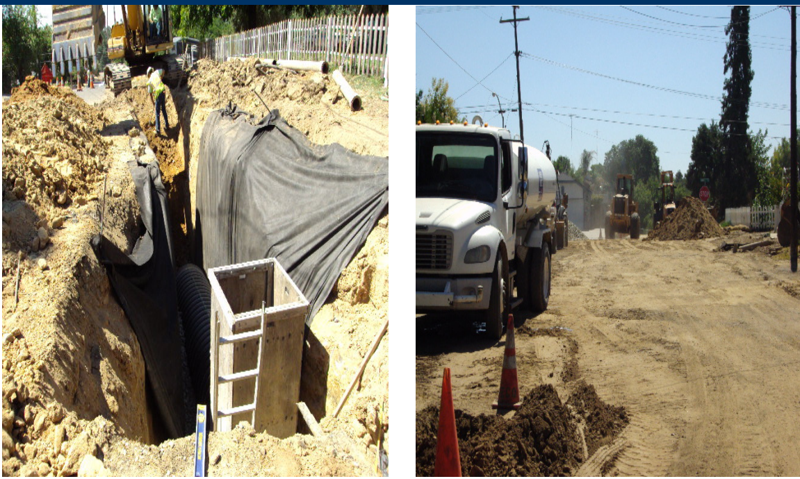
Photos reflect C and Covey Streets construction underground work in progress.
