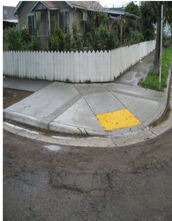
Photos reflect 3 rd Street ADA accessible ramp installations.
