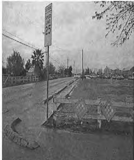
Photos reflect the Hoyer Road in need of curb, gutter, storm drain, sidewalk, ADA ramps and incidental street repaving.
