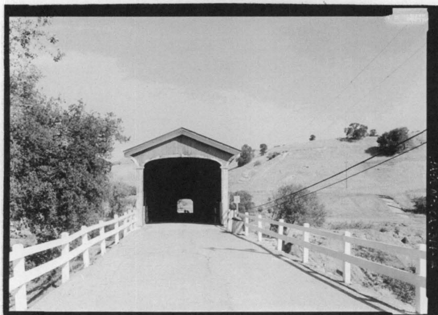
KNIGHT'S FERRY BRIDGE. Southeast portal elevation. Photograph by Jet Lowe, 2004 [HAER No. CA-314-2]
