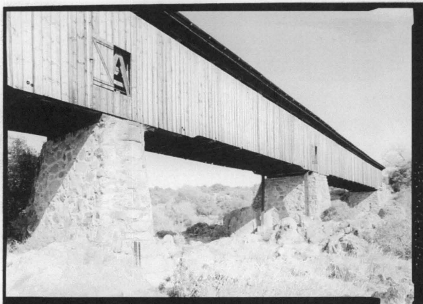
KNIGHT'S FERRY BRIDGE. Perspective view to southeast from midstream pier. Photograph by Jet Lowe, 2004 [HAER No. CA-314-13]
