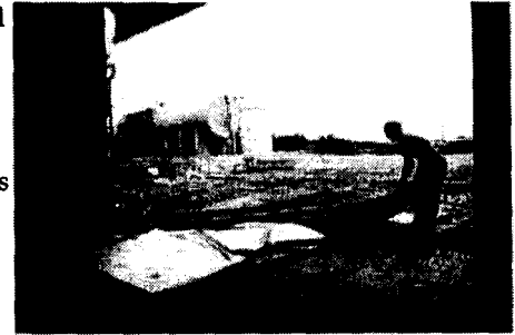
BART AH YOU/bahyou@modbee.com - A man who didn't want to give his name disassembles the old Indalex Inc. aluminum plant in north Modesto for scrap metal, says he can make up to $150 a day. October 10, 2011 - -
