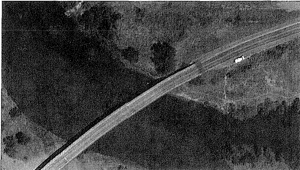
Aerial View of the bridge
