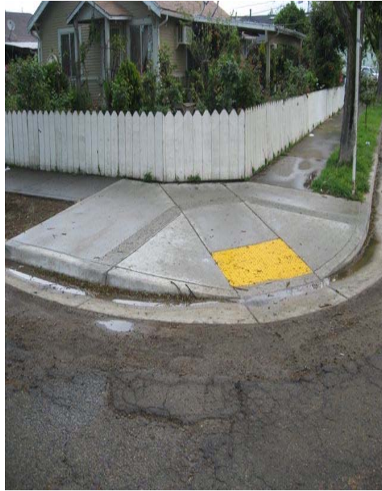
Photos reflect 3 rd Street where water main replacements were performed as well as installation of curb, gutter, storm drain, sidewalk and ADA accessible ramps.
