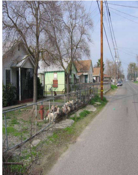
Photos reflect downtown residential streets lacking curb, gutter, storm drain, sidewalks, and ADA ramps in Ceres.
