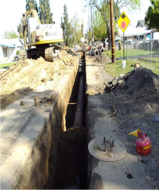
Photos reflect the installation of storm drainage and ADA curb cut improvements in Empire.
