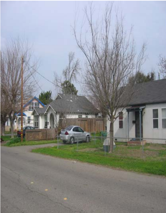
Photos reflect downtown residential streets lacking curb, gutter, storm drain, sidewalks, and ADA ramps in Ceres.
