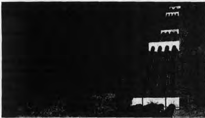
SAN FRANCISCO PUBLIC UTILITIES COMMISSION
