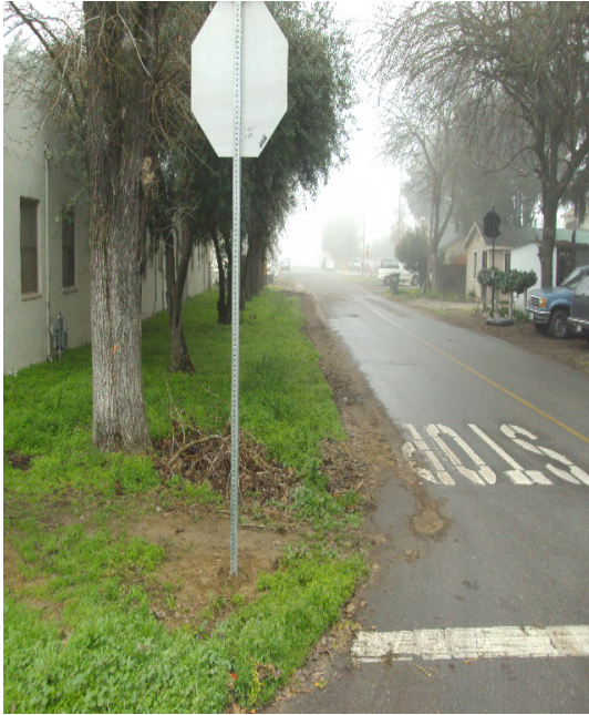
Photos reflect the need for infrastructure improvements such as curb, gutter, storm drain and ADA curb cuts along Pine Street, between 4 th and 7 th Streets.
