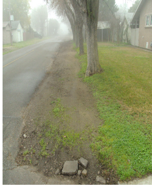
Photos reflect the need for infrastructure improvements such as curb, gutter, storm drain and ADA curb cuts along Pine Street, between 4 th and 7 th Streets.
