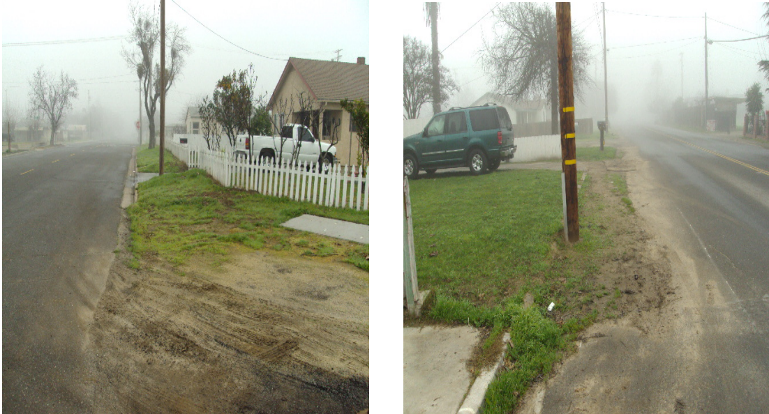
Photos reflect the need for infrastructure improvements such as curb, gutter, storm drain and ADA curb cuts in the area of Magnolia (from Central Ave. to El Camino St) and Don Pedro Road.
