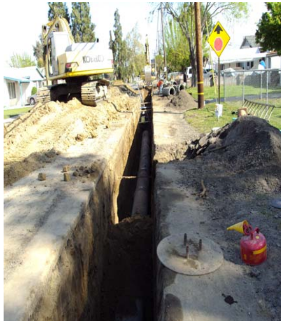
Photos reflect the installation of storm drainage and ADA curb cut improvements.
