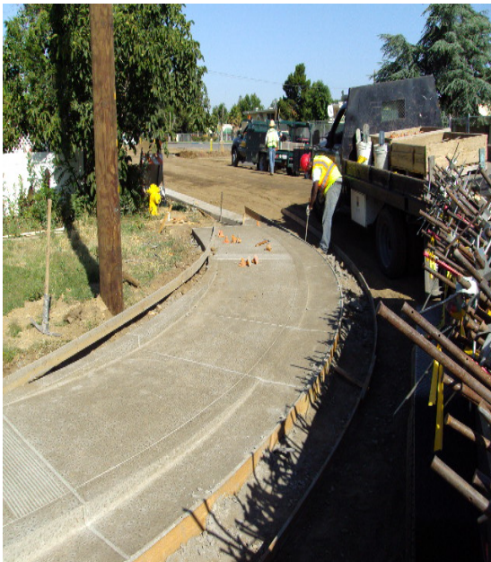
Photos reflect the installation of storm drainage and ADA curb cut improvements.
