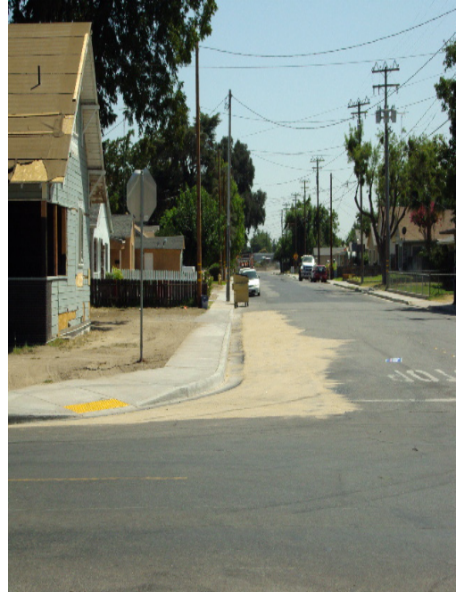
Photos reflect gutter, sidewalks, ADA ramps, and matching pavement improvements
