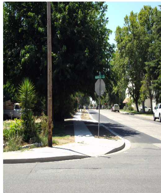
Photos reflect gutter, sidewalks, ADA accessible ramps, and matching pavement improvements.
