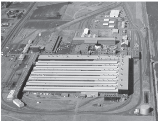
Riverbank Industrial Complex
