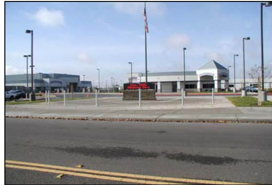
Full street frontage improvements
