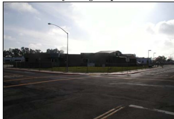
Full street frontage improvements
