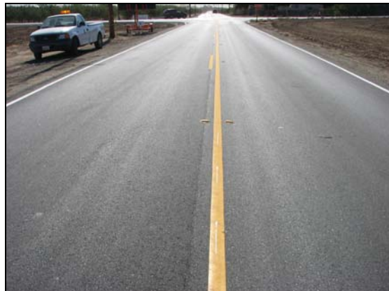
Marshall Road (Before and After)
