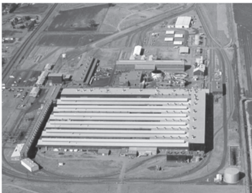
Riverbank Industrial Complex
